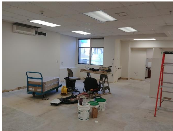
Division office, during the reno...2019
